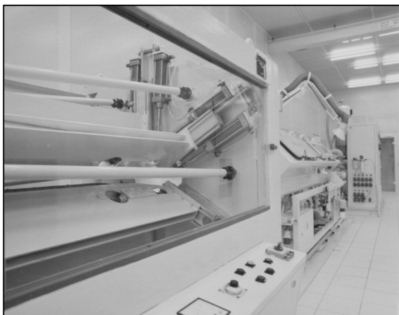
Figura 8 – Unità di estrusione tubi PVDF-UHP in camera bianca Figure 8 – Pipe extruder unit for PVDF-UHP production in clean room
